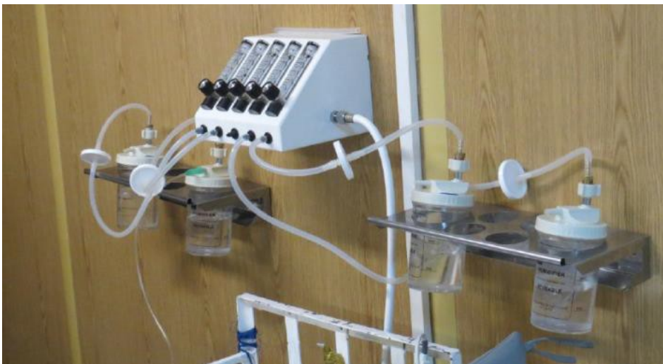
Figure 1: Circular antibacterial filters attached between the flow splitter and each humidifier. This is not necessary unless the patients are infectious by air transmission (e.g. tuberculosis).
