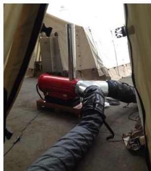
Example of a hybrid solution for tents (mechanic vent for air IN and OUT + UVGI light treatment)
